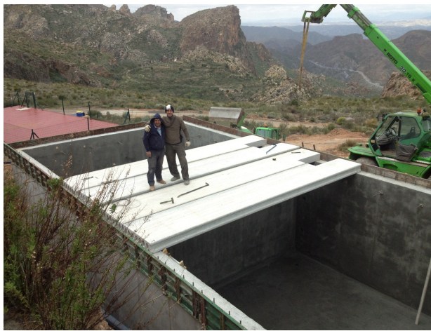
Concrete Shell Water Deposit (Sopalmó Road)
